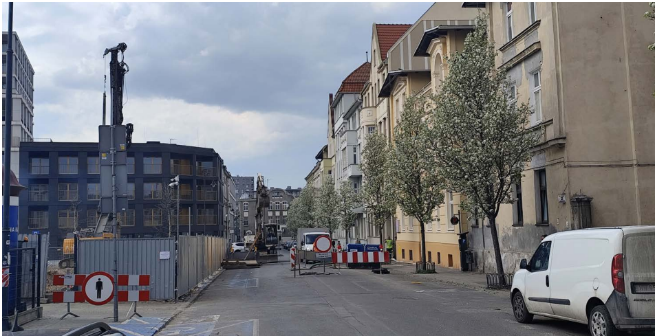
Figure 5: Traffic disruption at a housing construction site (SAFE project).
